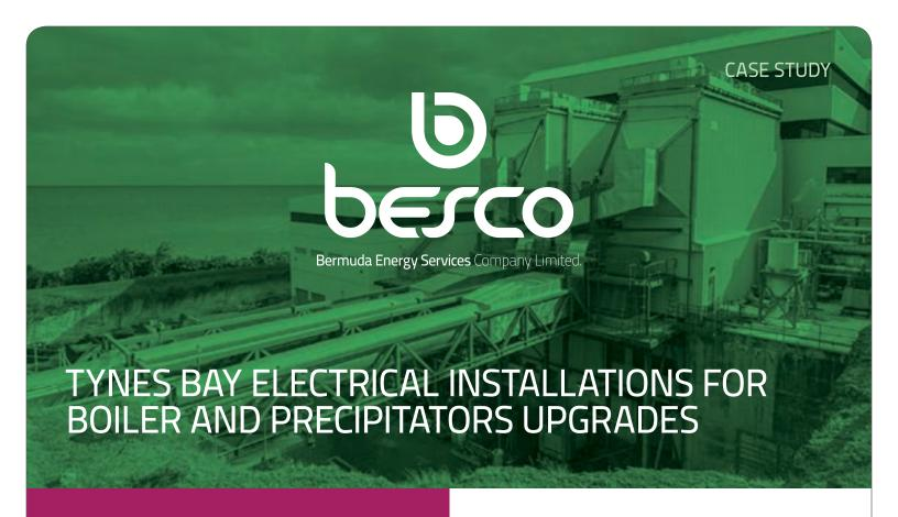
The Tynes Bay Waste Treatment Facility incinerates Bermuda's domestic waste through two separate waste processing streams. The incineration process reduces the Island's volume of combustible waste and replaces the old land fill facility at Marsh Folly. A secondary function of the Tynes Bay waste incineration process is to extract the energy produced by the combustion gasses to produce steam and then convert to electric power.
